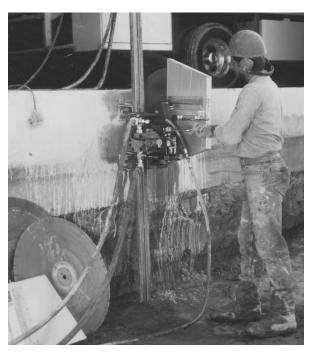
Illustration 16 - Securely mounted wall saw
